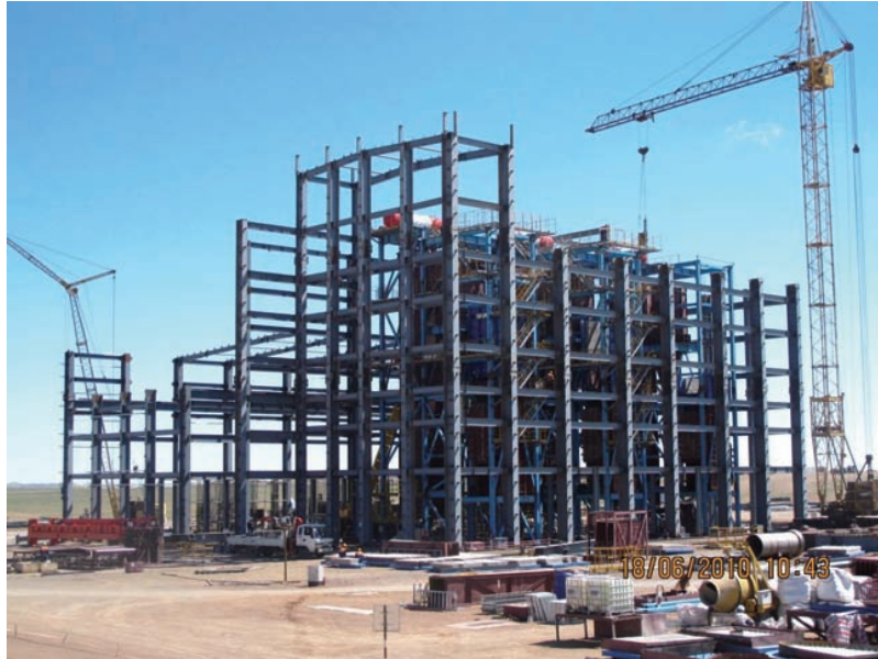
Photo 4.3 Power Plant Construction
