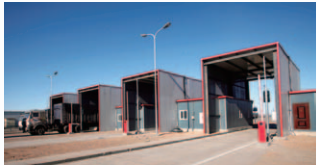
GS border crossing check point expansion
