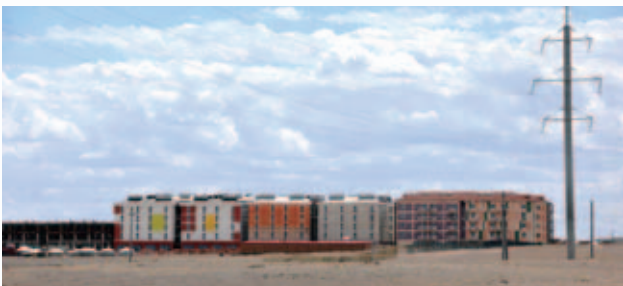
MMC's housing project in Tsogttsetsii soum
