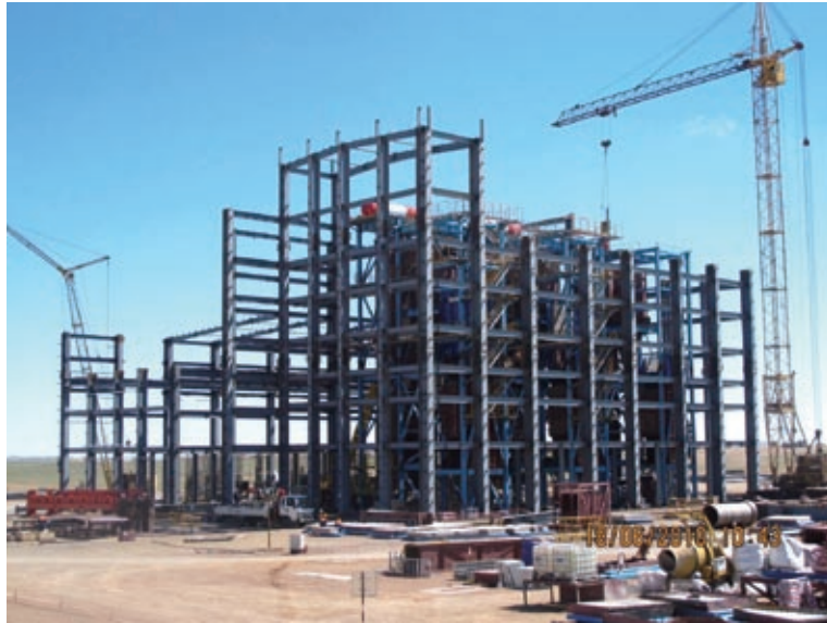
Photo 4.3 Power Plant Construction
