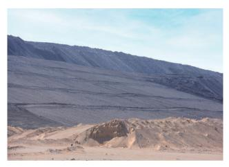
During technical rehabilitation: Covering topsoil on the shaped waste piles.
