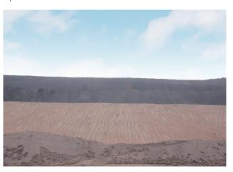
From 2020 to 2022, three hectares of waste dump were sloped, shaped, and planted with vegetation. Maintenance and protection of this area were managed by a professional organisation. Replanting work was carried out from July to August 2023, on the sections where vegetation growth was not progressing well.
